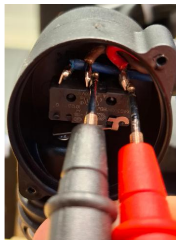
Check the pressure switch
